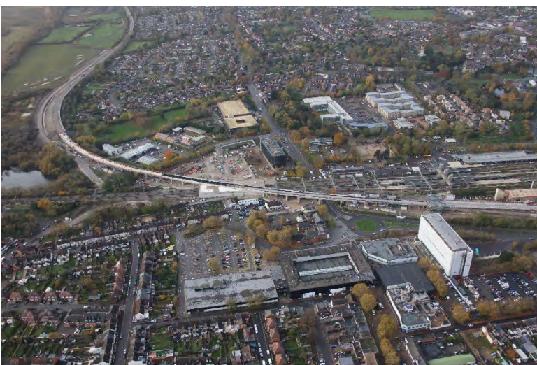
Bletchley Flyover structural competition, November 2021. Image courtesy of Network Rail Air Ops
